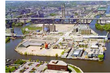
Aerial View looking west for the proposed site at 6th and Canal Streets for the Harley-Davidson Museum
